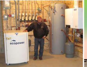
Large Residential (> 7,000 ft<sup>2</sup>), light commercialheat is primary focus with electrical generation maximized for off-set of electric costs. 3- 10kW. Installed costs now: \$35-\$45,000, Tgt: < \$20-\$25,000 Maintenance costs: \$6-\$800/yr.
