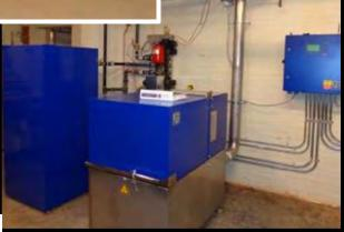
Light Commercial-- Primary focus is maximum heat production, with offset of power costs. 12- 30kW. Installed costs now: \$3- \$4,000/kW. Target is: \$2,000/kW. Maintenance: \$8-\$1K/yr
